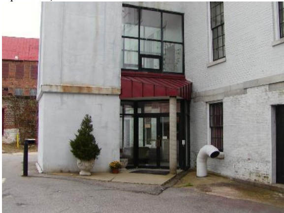
Figure 1.12: West Elevation, Siege Museum. (Photograph 8/10 October 2004)
