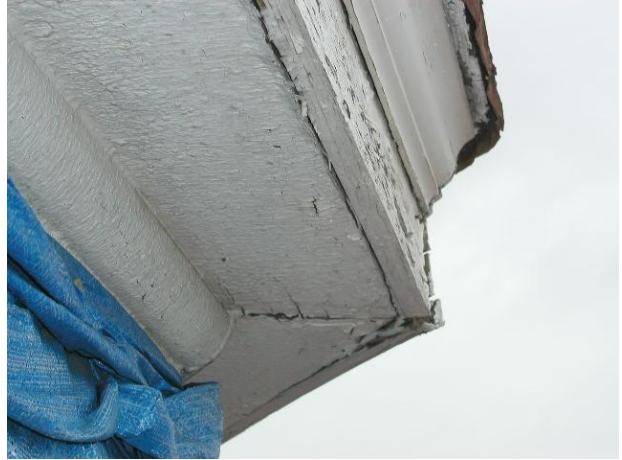
Photo No. 16 General observation of wood and paint finishes.
