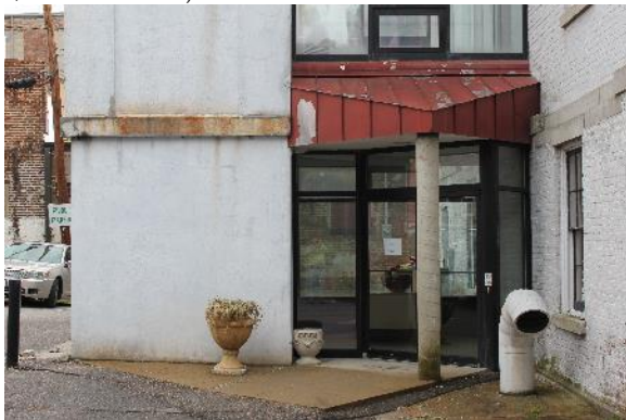
Figure 1.13: West Elevation, Siege Museum(Photograph 7 April 2015)
