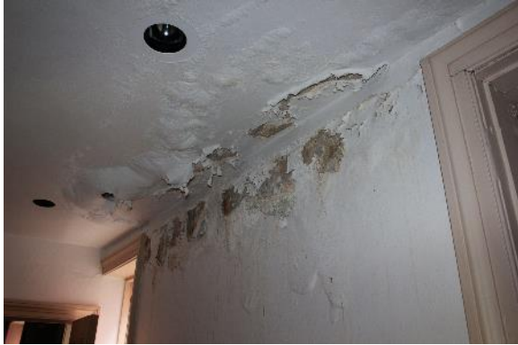
Figure 1.32: Ground floor, Siege Museum. (Photograph 7 April 2015)
