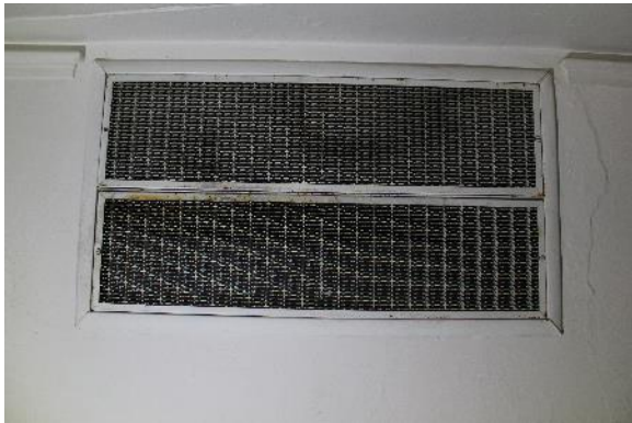
Figure 1.22: Second floor, Siege Museum. (Photograph 7 April 2015)
