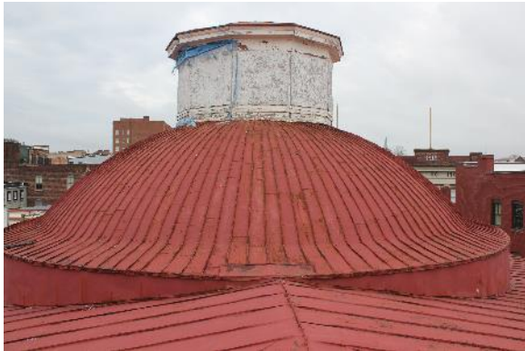
Figure 1.1: Roof, Siege Museum. Dome roof and cupola. (Photograph 7 April 2015)
