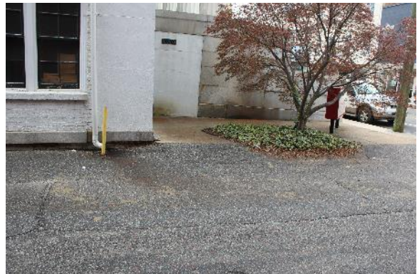
Figure 1.10: West Elevation, Siege Museum. (Photograph 7 April 2015)
