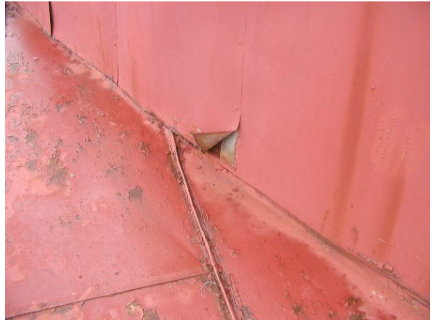
Photo No. 13 Observation - light gauge panel material noted. Painted and unpainted surfaces noted.
