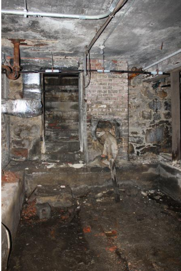
Figure 1.37: Basement, Siege Museum. (Photograph 7 April 2015)
