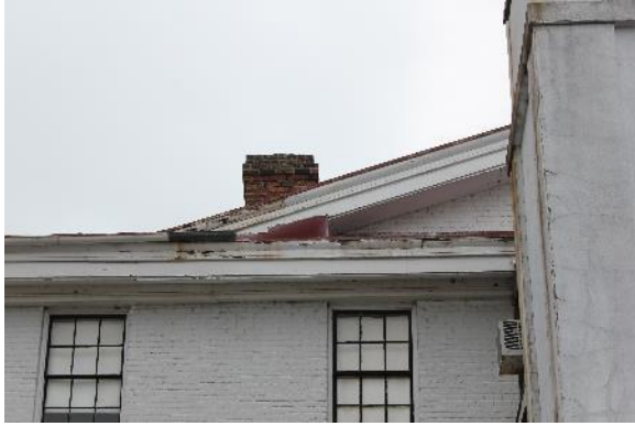
Figure 1.18: North Elevation, Siege Museum. Cornice Detail. (Photograph 7 April 2015)
