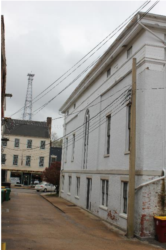
Figure 1.7: East Elevation, Siege Museum. Cornice Detail. (Photograph 7 April 2015)
