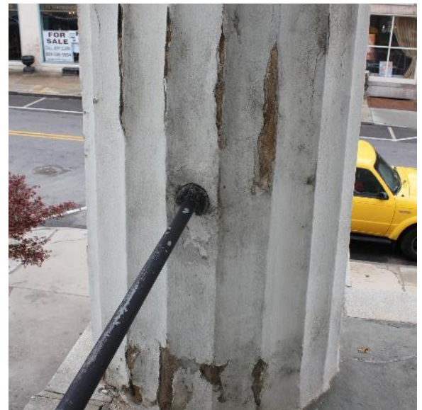
Figure 1.6: South Elevation, Siege Museum. Handrail detail. (Photograph 7 April 2015)
