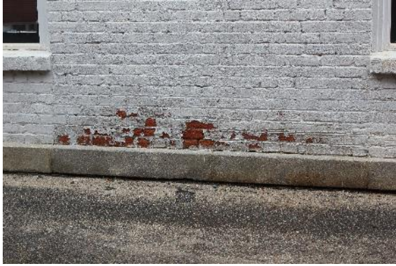
Figure 1.11: West Elevation, Siege Museum. (Photograph 7 April 2015)
