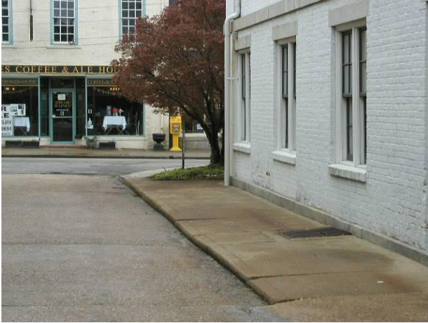
Photo No. 33 Observation – front corner downspout routed to below grade storm sewer.
