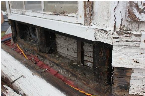
Figure 1.2: Roof, Siege Museum. Cupola wall cavity detail. (Photograph 7 April 2015)
