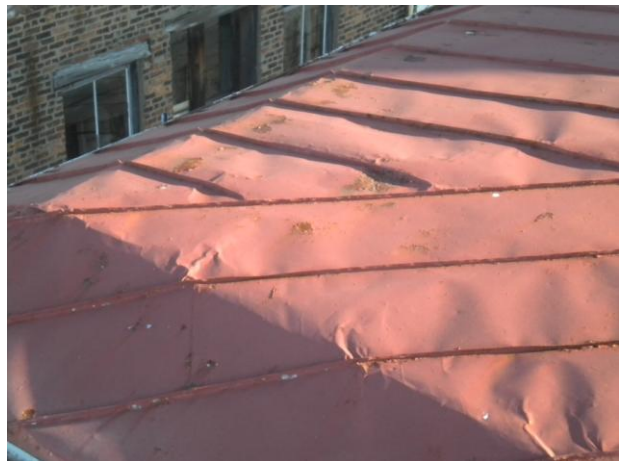
Photo no. 20 Observation – transition in perimeter deck slope.
